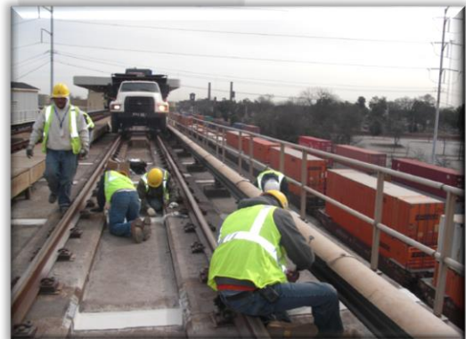
MARTA Grout Pockets - Heavy Construction
