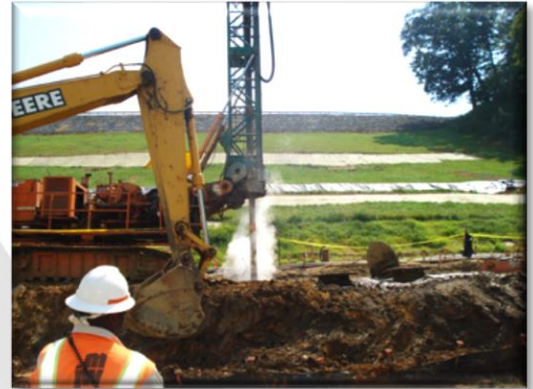
Blue Ridge Dam - Blue Ridge, Georgia
