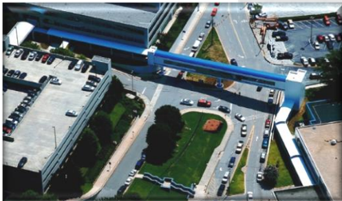
Decatur VA Pedestrian Bridge - Decatur, GA
