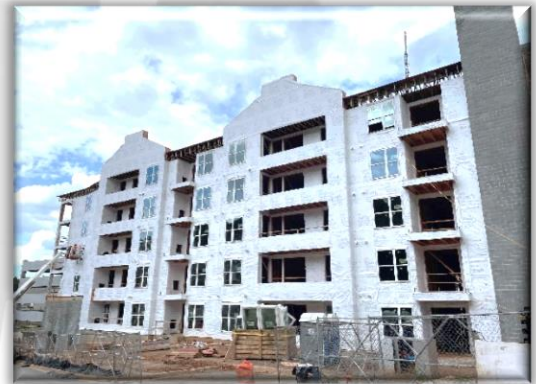
Avondale Hills - New Construction
