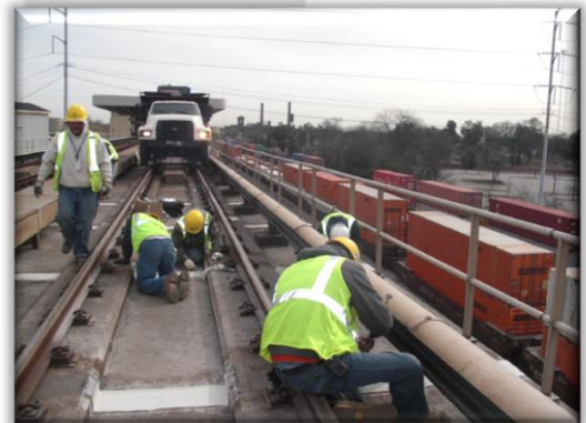
MARTA Grout Pockets - Heavy Construction
