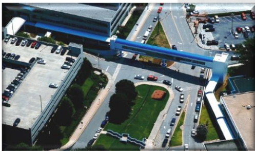
Decatur VA Pedestrian Bridge - Decatur, GA
