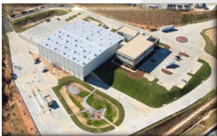
DeKalb County Transfer Station - Atlanta, GA
