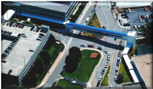
Decatur VA Pedestrian Bridge - Decatur, GA
