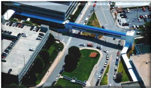
Decatur VA Pedestrian Bridge - Decatur, GA
