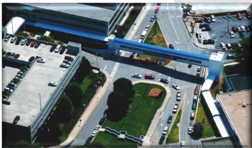
Decatur VA Pedestrian Bridge - Decatur, GA
