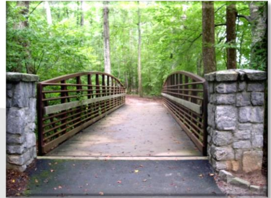
Jones Bridge Park - Gwinnett County, Georgia
