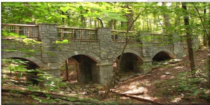
Deepdene Park Restoration - Atlanta, GA
