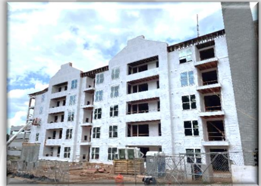
Avondale Hills - New Construction
