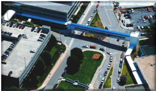
Decatur VA Pedestrian Bridge - Decatur, GA
