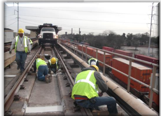
MARTA Grout Pockets - Heavy Construction
