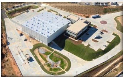
DeKalb County Transfer Station - Atlanta, GA
