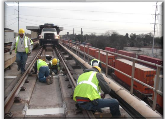
MARTA Grout Pockets - Heavy Construction
