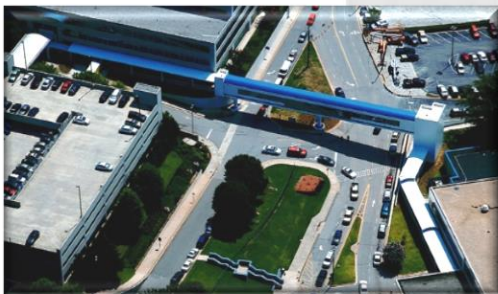
Decatur VA Pedestrian Bridge - Decatur, GA
