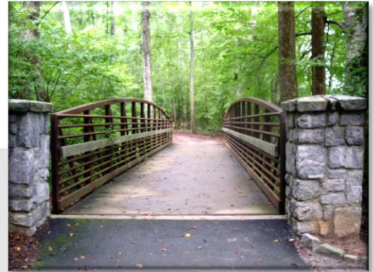
Jones Bridge Park - Gwinnett County, Georgia
