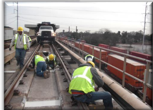
MARTA Grout Pockets - Heavy Construction
