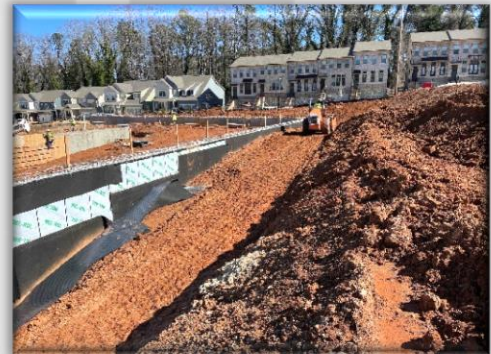
Avondale Hills - New Construction
