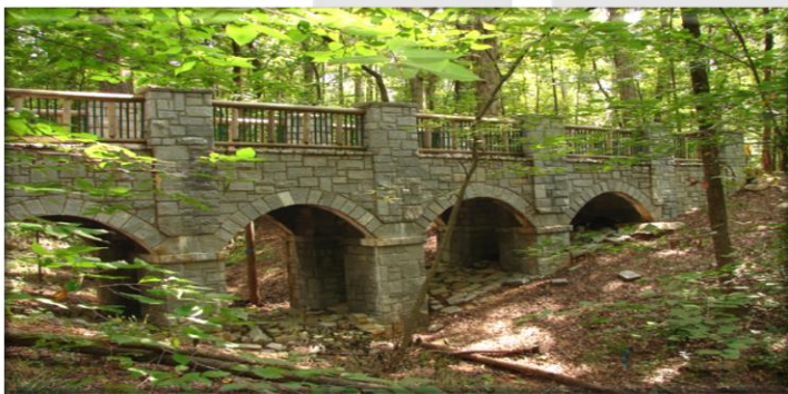
Deepdene Park Restoration - Atlanta, GA
