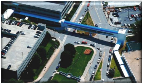
Decatur VA Pedestrian Bridge - Decatur, GA
