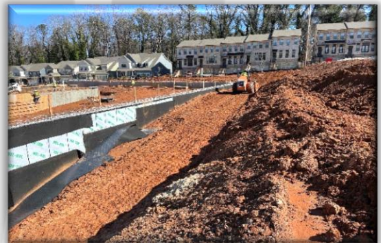
Avondale Hills - New Construction
