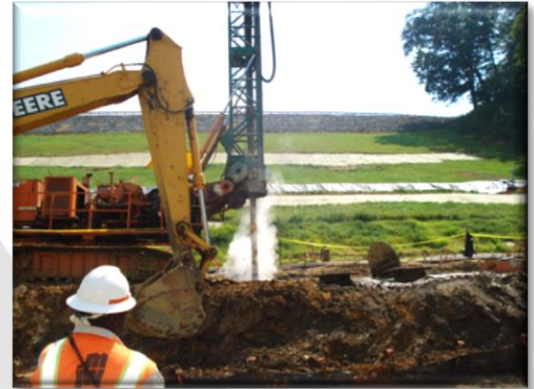
Blue Ridge Dam - Blue Ridge, Georgia
