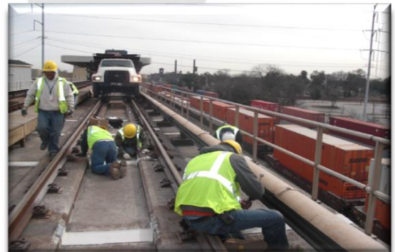
MARTA Grout Pockets - Heavy Construction
