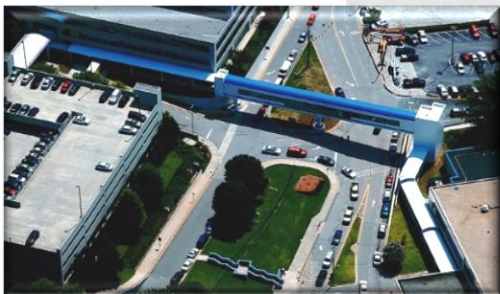
Decatur VA Pedestrian Bridge - Decatur, GA
