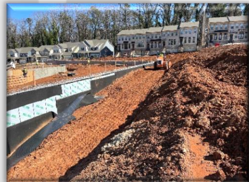
Avondale Hills - New Construction
