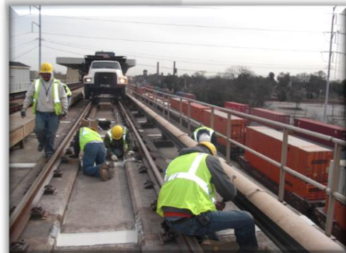
MARTA Grout Pockets - Heavy Construction
