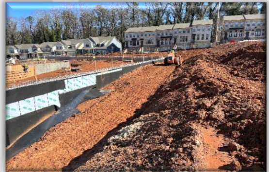
Avondale Hills - New Construction
