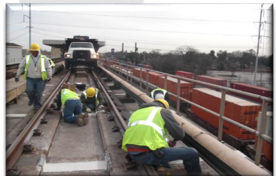
MARTA Grout Pockets - Heavy Construction
