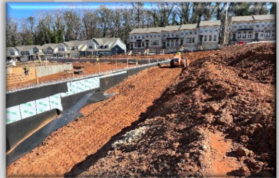
Avondale Hills - New Construction
