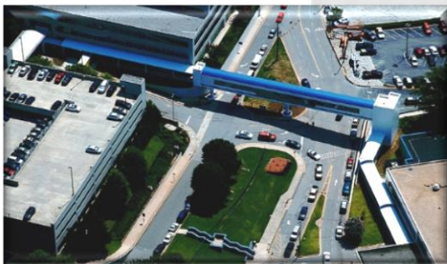
Decatur VA Pedestrian Bridge - Decatur, GA
