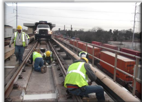
MARTA Grout Pockets - Heavy Construction
