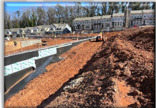
Avondale Hills - New Construction
